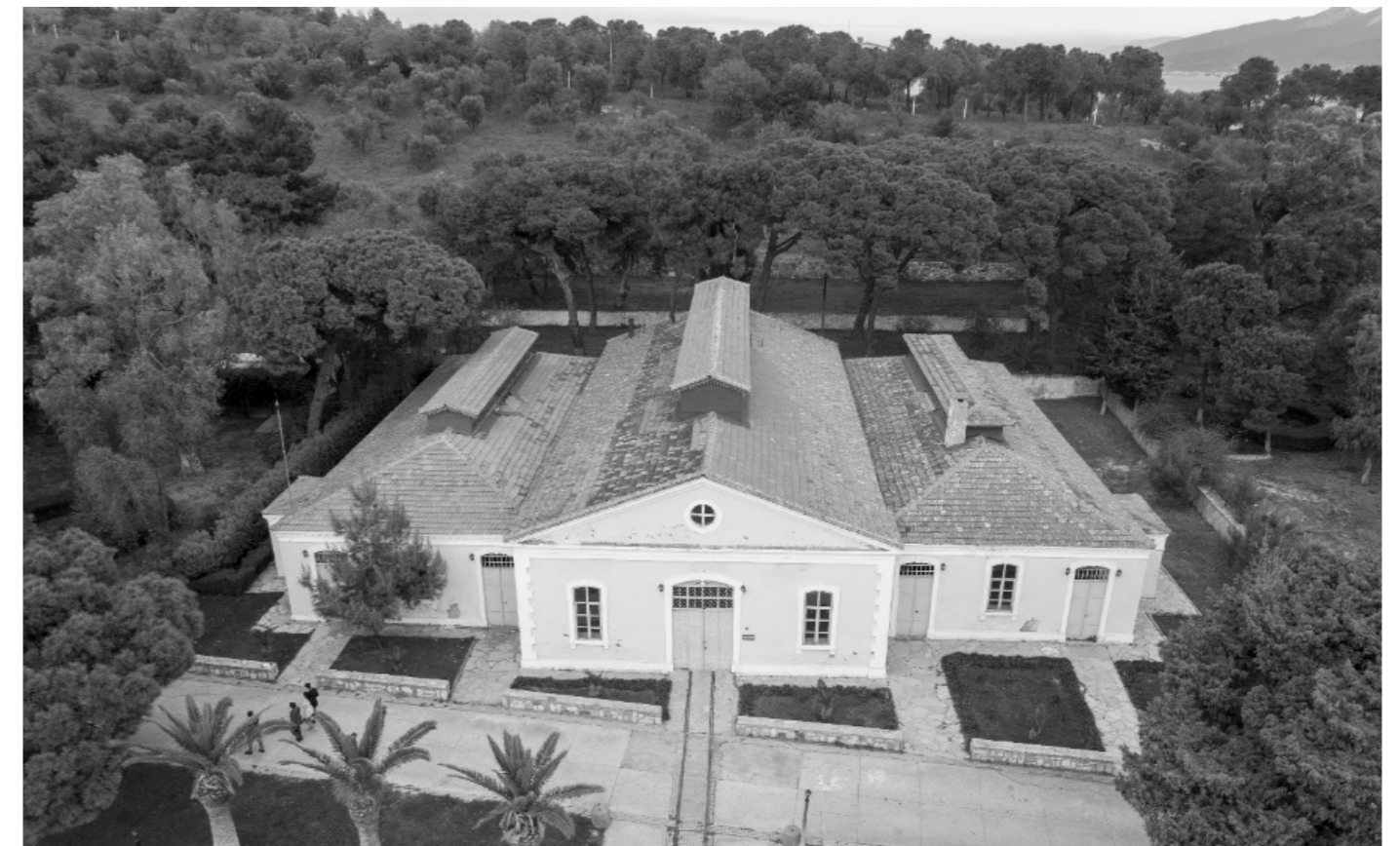
Figure 17. The main entrance of the station with the railway, Urla Quarantine Island. Source: Turkey Ministry of Health General Directorate of Border and Coastal Health in Urla, taken by author.
