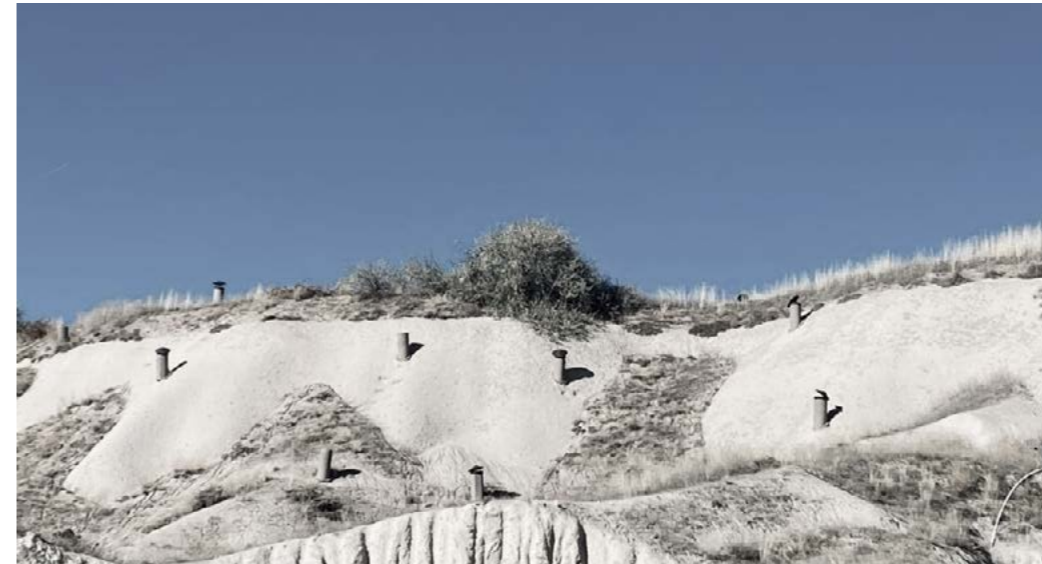
Figure 10. Exterior view of "potato storages" with chimneys in Cappadocia, 2022, taken by İdil Bilici.
